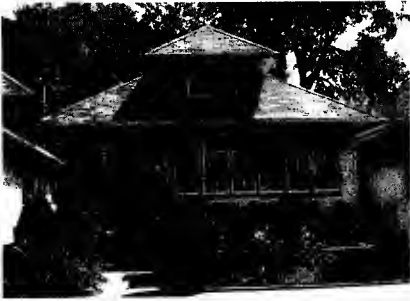
Figure 1: 7641 South Merrill Avenue
